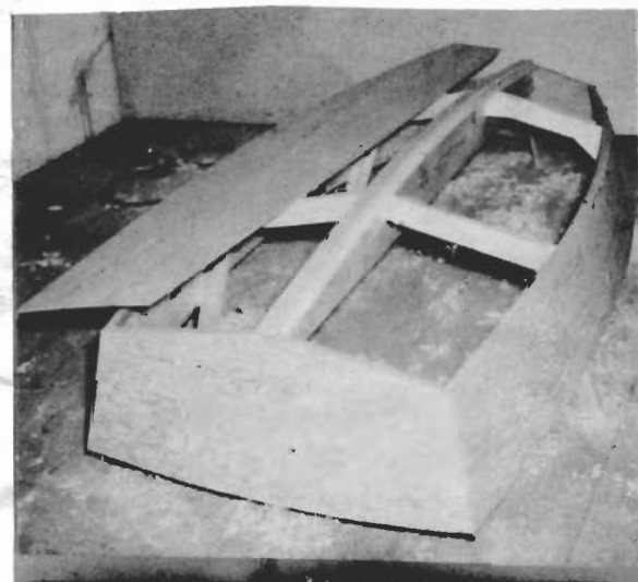
Outer keel in place -- sides trimmed at transoms.
